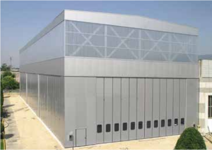
External view, folding doors with double leaf packs 6+6, with side fixed panels, height of the hole 8000mm
