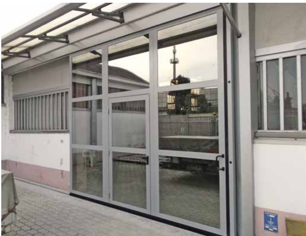
External view, sliding door with single leaf, with pedestrian door with lowered obstacle
