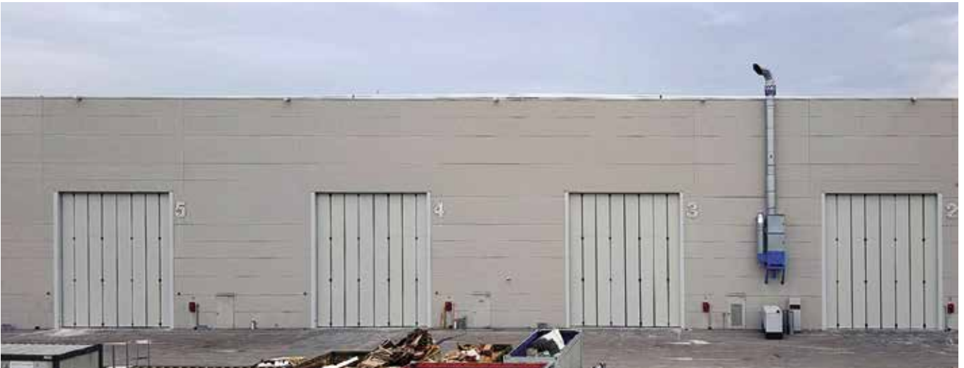
External view, folding door with double leaf packs 4+4, motorized, height of the hole 9000mm
