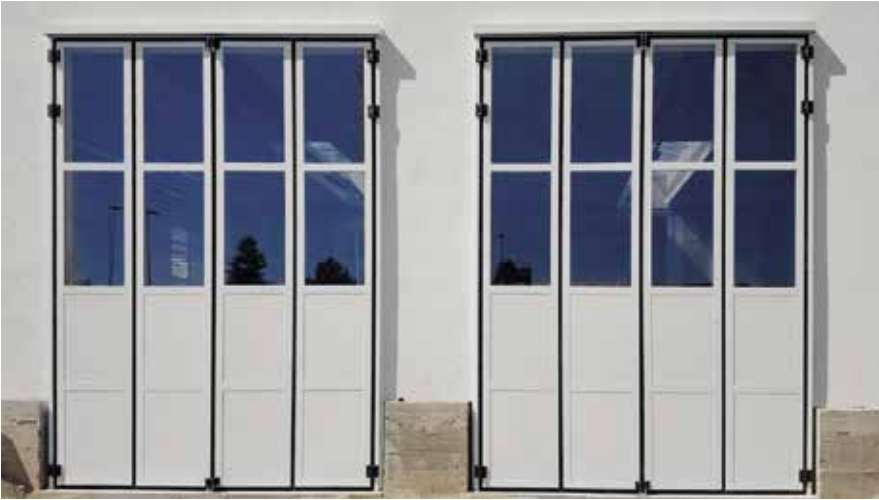
External view, door with duoble leaf packs, with iron grating welded
