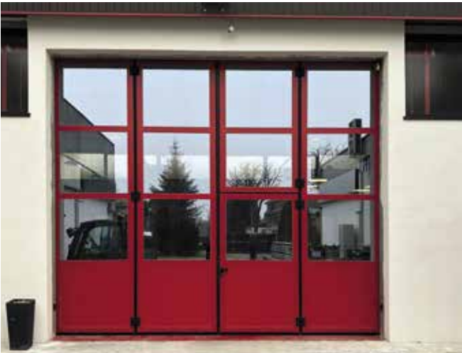
External view, door with duoble leaf packs 2+2, central broken leaf, motorized
