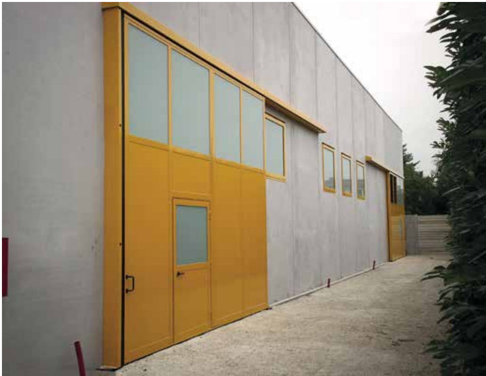
External view, sliding door with single leaf, with pedestrian door without obstacle
