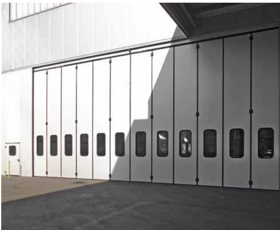
< Folding door with double leaf packs 8+8, motorized, height of the hole 7000mm
