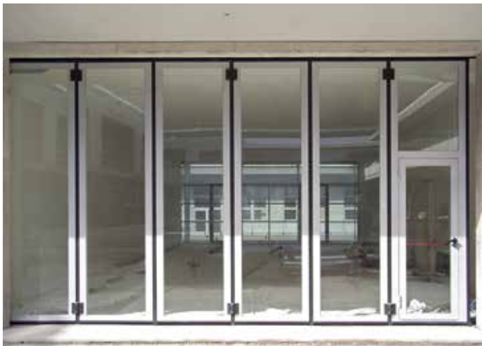
External view folding door with double leaf packs 6+6, motorized
