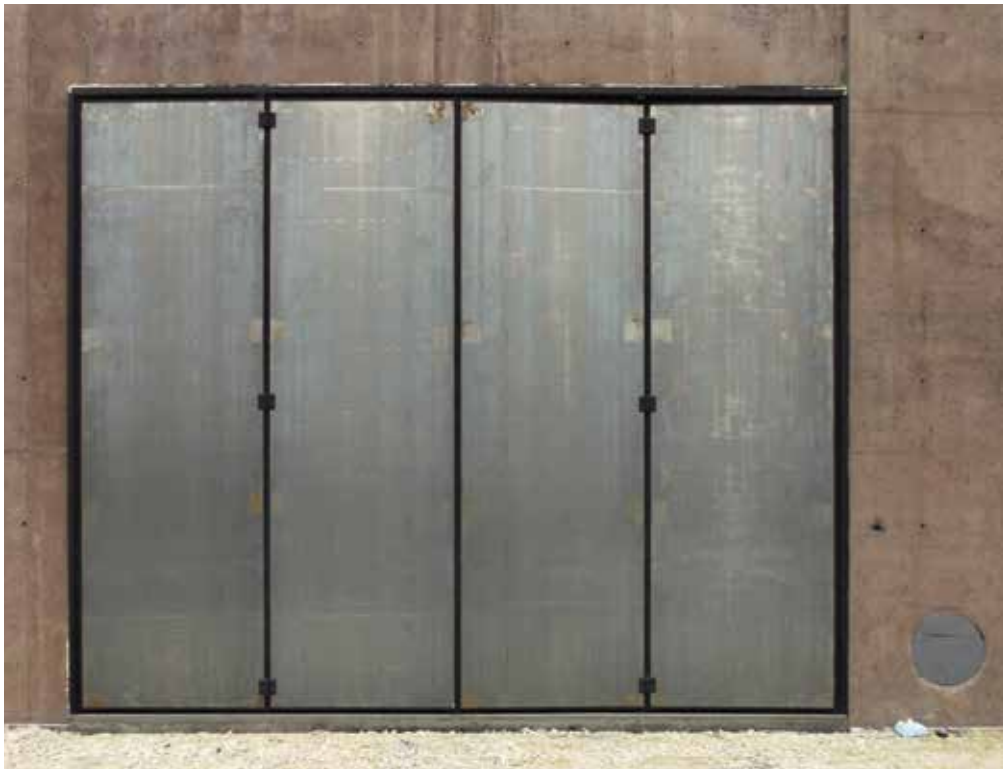
External view, folding door with double leaf packs 2+2, without track on floor, made with corten steel sheets
