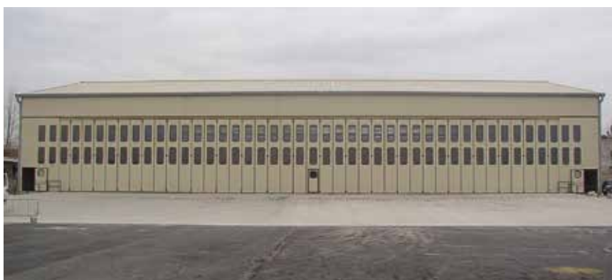
External view, doors with double leaf packs 20+20, with double row of portholes and motor
