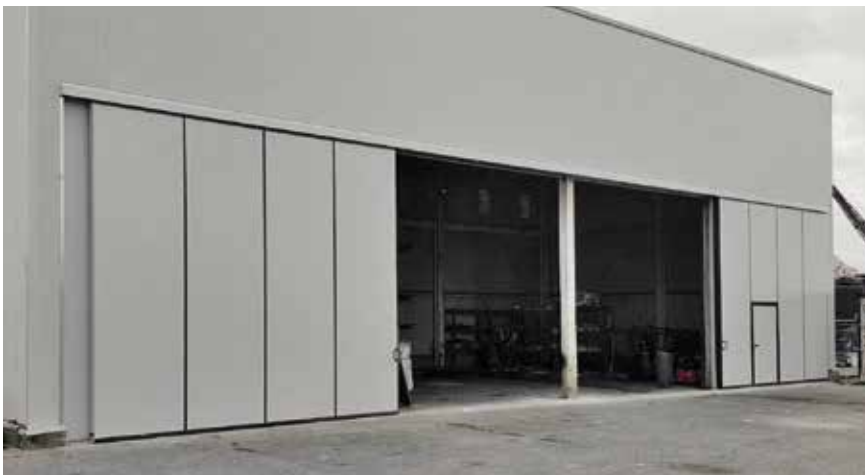
External view, sliding door with opposed double leaves, with pedestrian door with lowered obstacle
