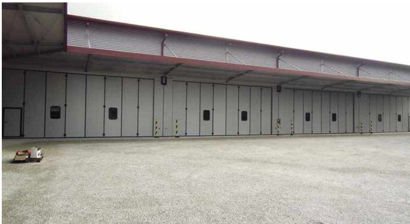
External view, doors with double leaf packs 4+4, motorized, with fixed side panels
