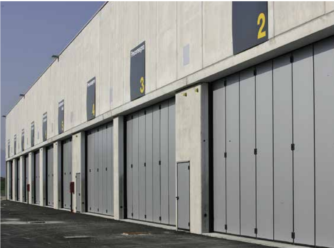
External view, doors with double leaf packs 8+8, with portholes and motor
